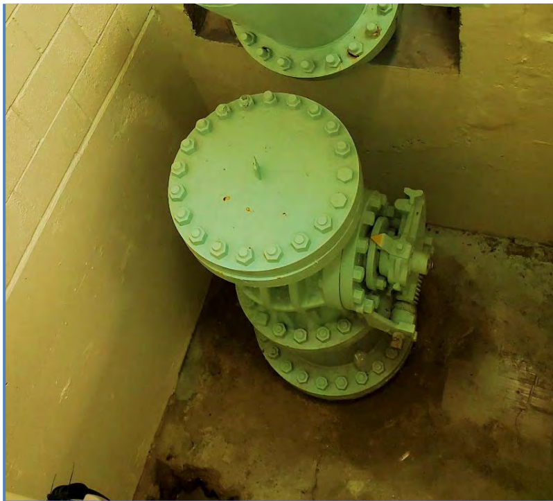
Figure 7.6 – Typical Service Connection/Outlet Nozzle (Blind Flanged as Shown)
