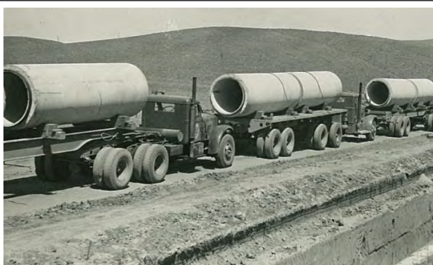
Early San Diego County pipeline segments
