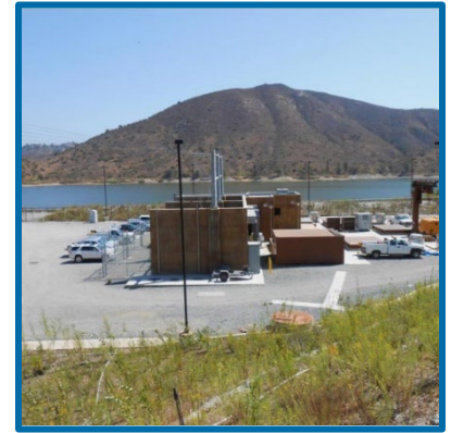
Lake Hodges Projects $208 million
