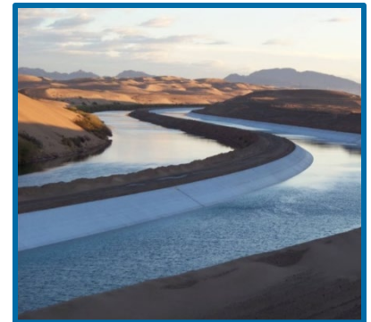
All-American & Coachella Canal Lining Project $447 million ($190 million from Water Authority)
