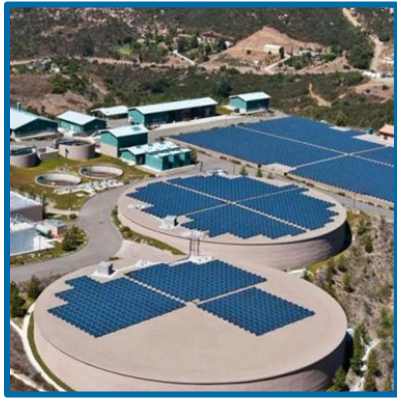
Twin Oaks Valley Water Treatment Plant $179 million
