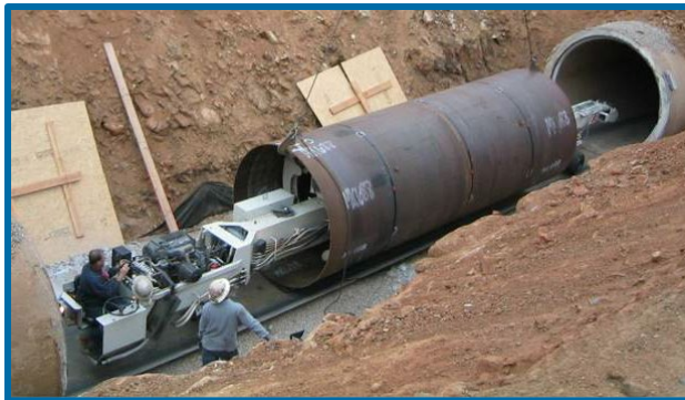
Pipeline Relining $493 million
