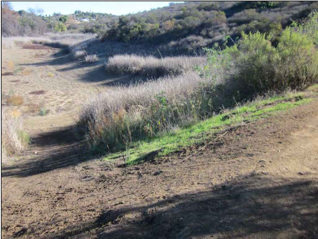
Figure 6. The earthen dam and reservoir, facing north east.
