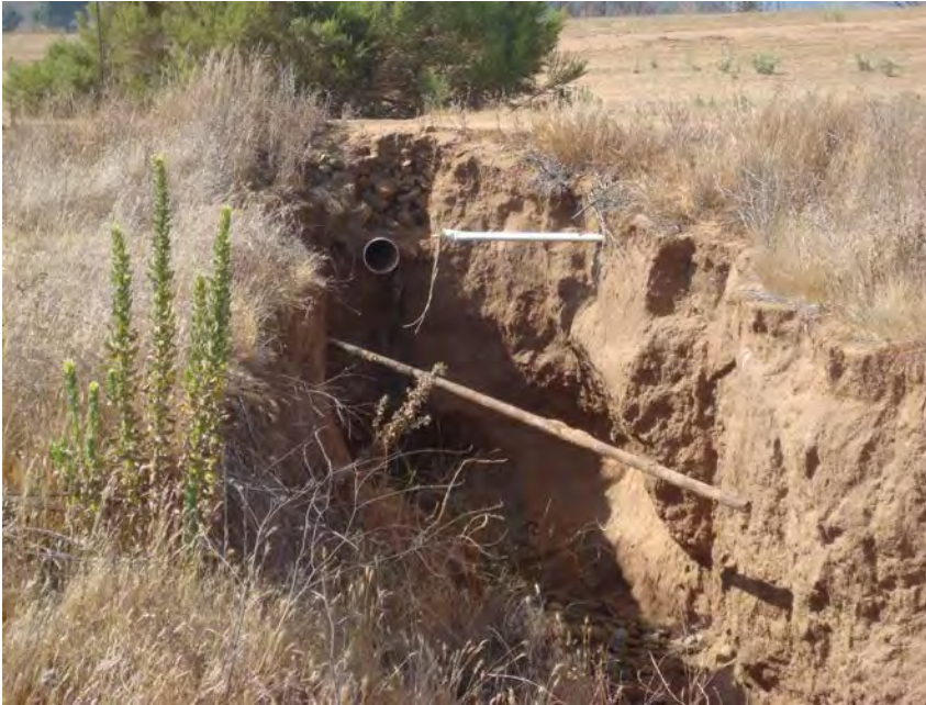
View of drainage trench and piping, facing north.
