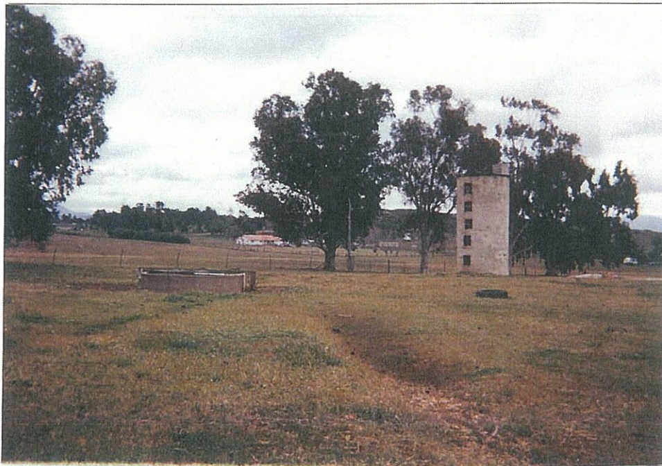
2. Grain silo and watering hole across driveway from main residence. View to the east, includes pasture land along the southern property boundary.
